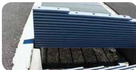
These grating panels are installed as a trench cover for a system that can charge electric vehicles in motion.
