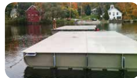
Five foam-filled fiberglass rafts support a timber deck and walkways designed for a 12-ton vehicle.
