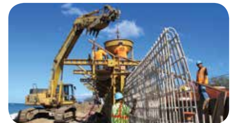
Pultruded glass-reinforced composite rebar replaced epoxy steel in concrete.
